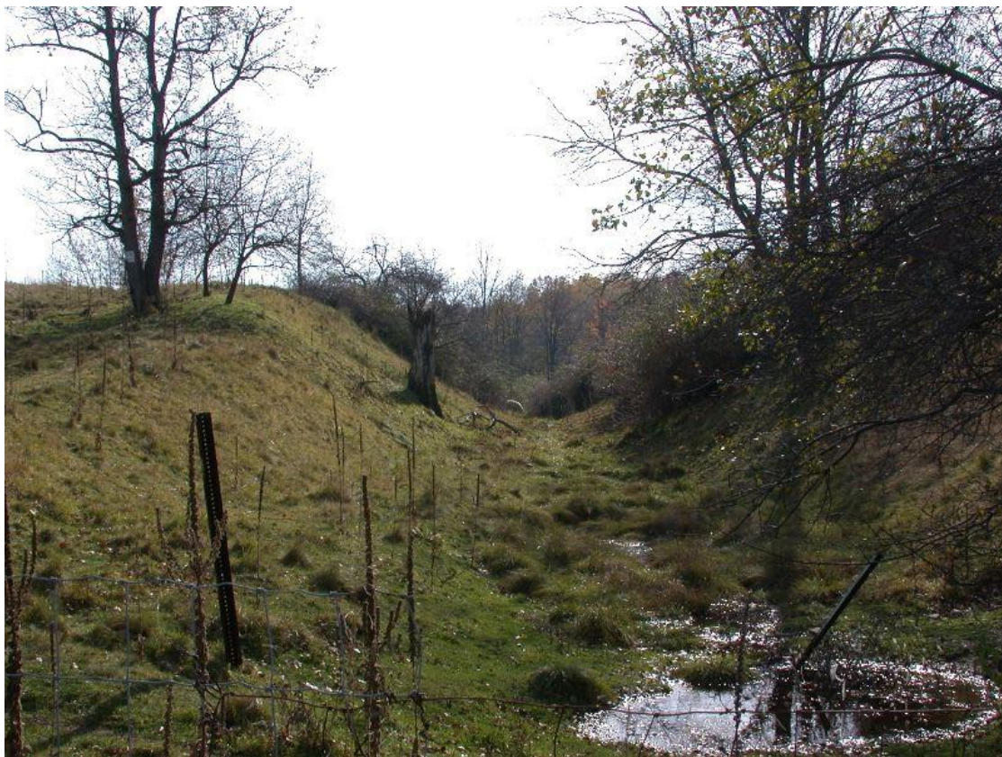
cut at Millard Hill Rd., facing S. 29-October-2003
